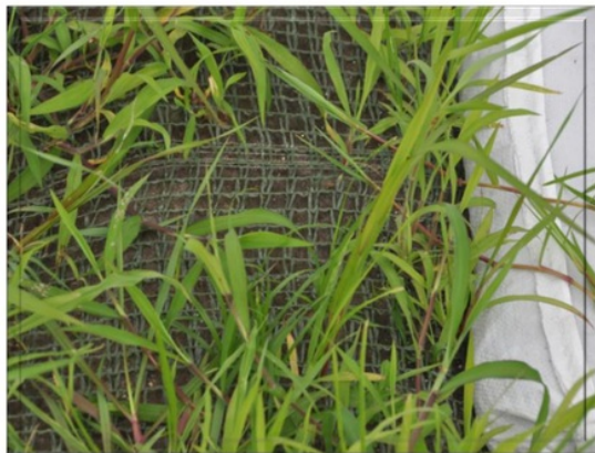
Figure 4. Erosion control mats in the Kamisaigo River.
